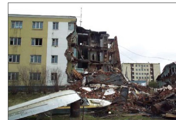
Damaged building caused by instability in foundation, Chersky settlement 2
